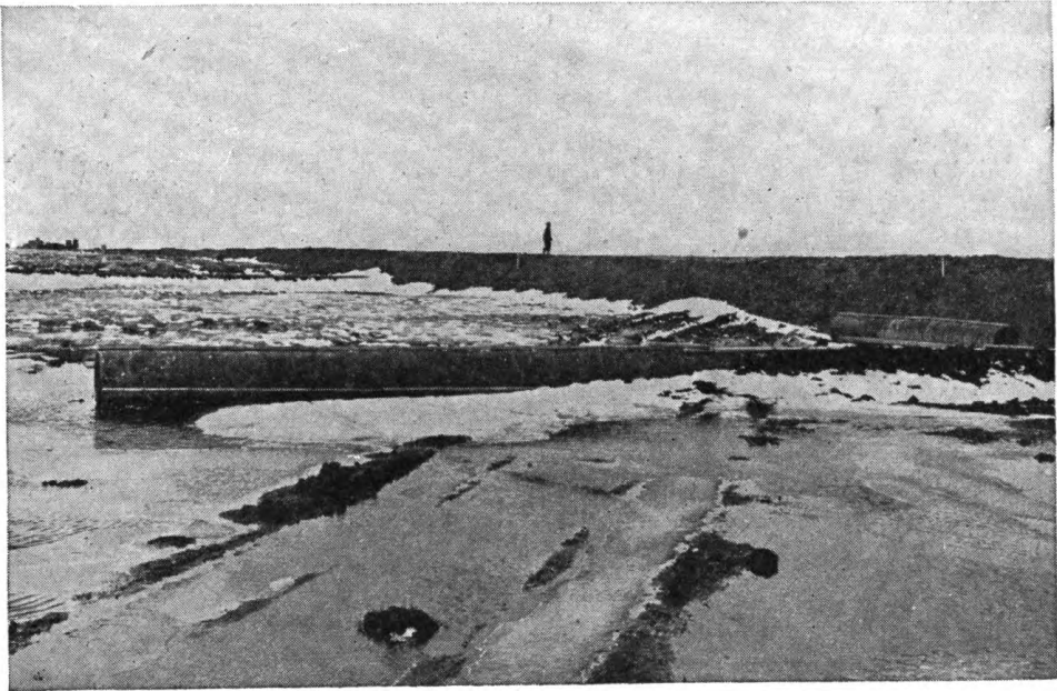
Figure 50. An expedient culvert made of oil drums.
